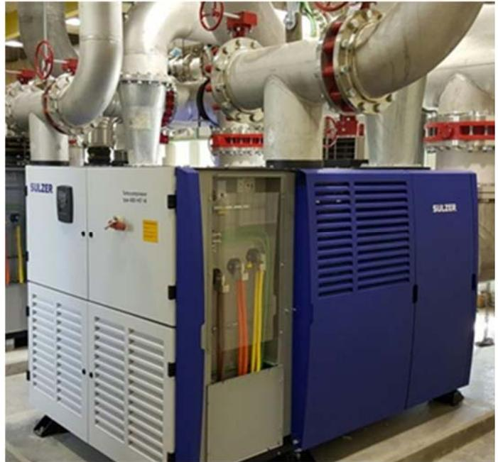
*New turbo blowers (manufactured by Sulzer-ABS).*
