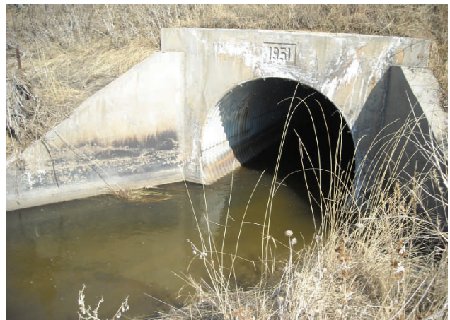
Union Pacific Railroad culvert near Colorado Blvd.
