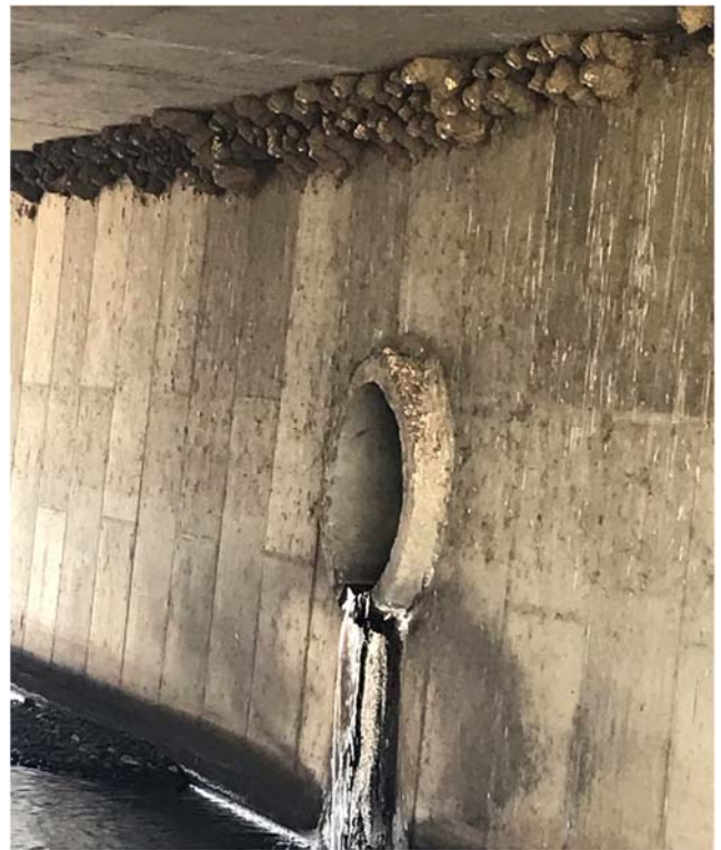
Dry weather flows from a storm drain under a bridge with swallow nests under the bridge deck. E. coli can originate from both human and natural sources.
