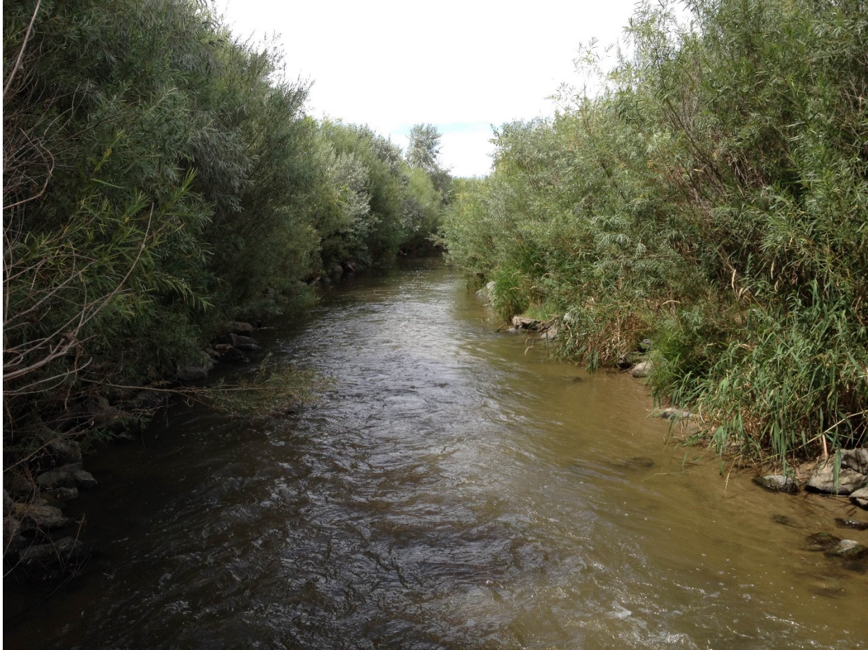
Photo 9, Reach 5A: This reach appears to have been stabilized with rip-rap along the bank toes and possible willow plantings. The channel bed in this section is primarily stiff clay which may slow further incision. The lack of alluvium also suggests this reach has an excess of transport capacity. View looking downstream.
