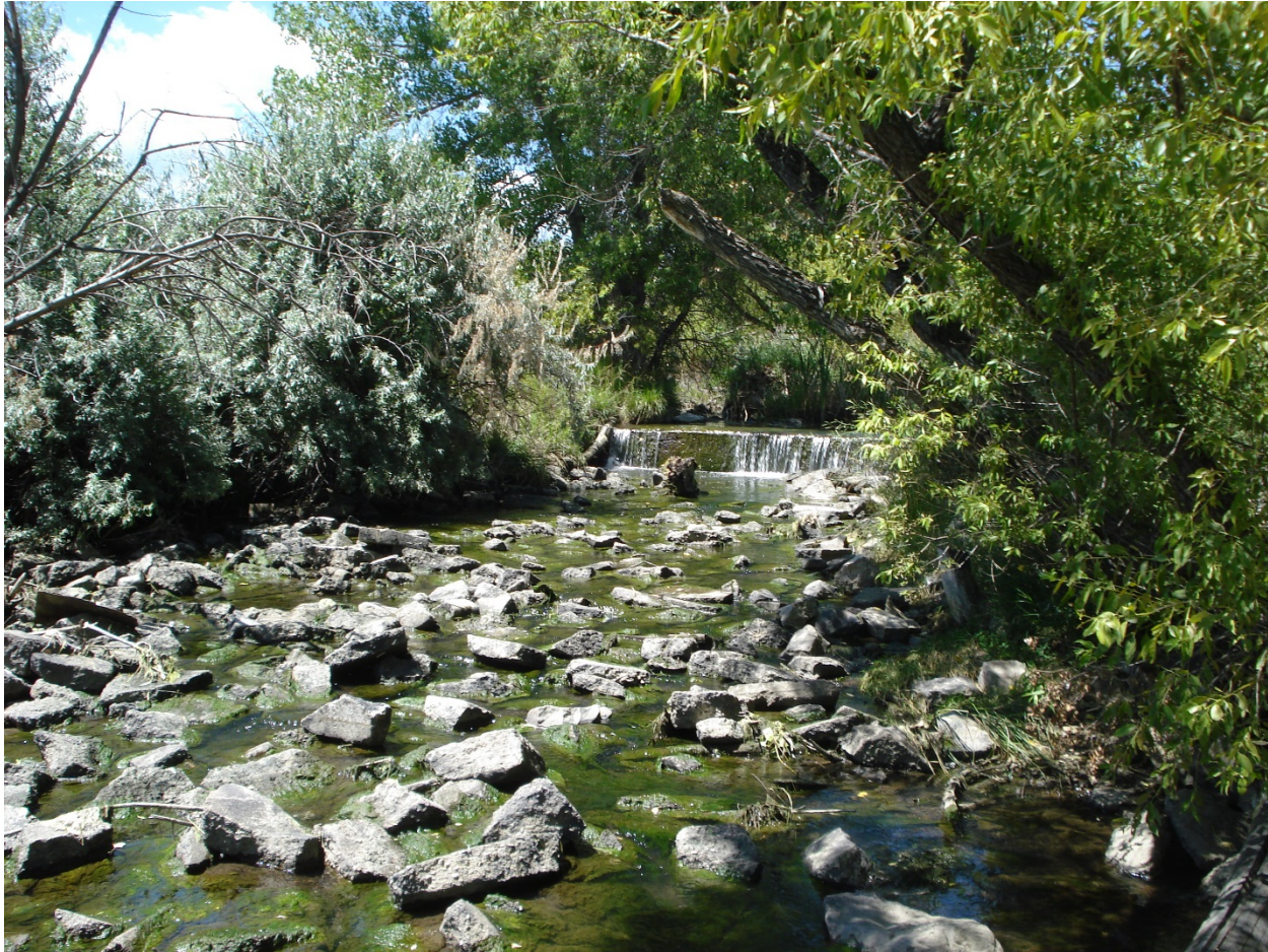
Photo 1, Reach 1C: Looking upstream at a grade control structure in the upper part of Big Dry Creek. Note significant amount of rip-rap downstream from structure stabilizing the bed. This substrate also provides structure for filamentous algae growth.
