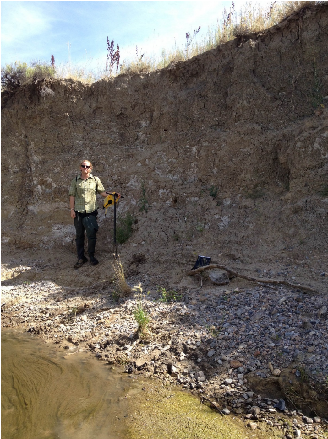
Photo 5, Reach 3C: A tall, nearly vertical cutbank (~ 4.5 m or 15 ft). Sparse vegetation is doing little to stabilize this bank. Flow direction is left to right.
