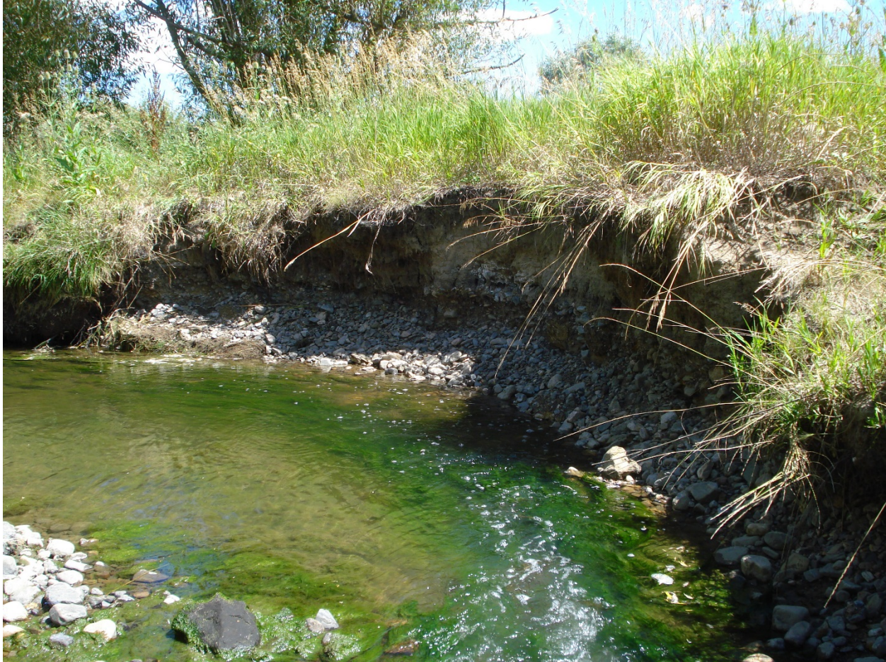
Photo 2, Reach 2A: An eroding bank on the outside of a meander bend. In this section of Big Dry Creek, there is still significant coarser bed material. This coarse material makes up the majority of the bank toe while the upper bank is all sandy clay. View looking downstream.
