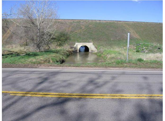
*Undersized culvert at the Union Pacific Railroad embankment near Colorado Blvd. provides inadvertent detention of flows in Big Dry Creek.*
